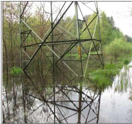
Figure 33 -Damages due to floodplains and subsidence - deviation from verticality (GIG's archives)
