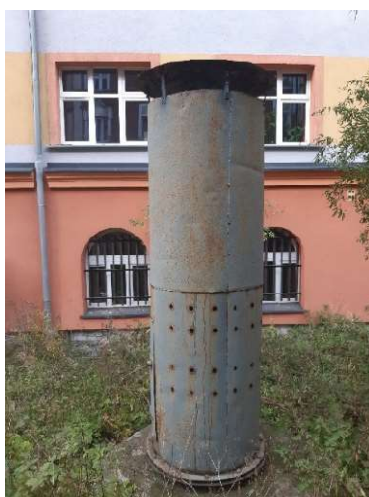
Figure 25 -Degassing well (M.Wysocka)
