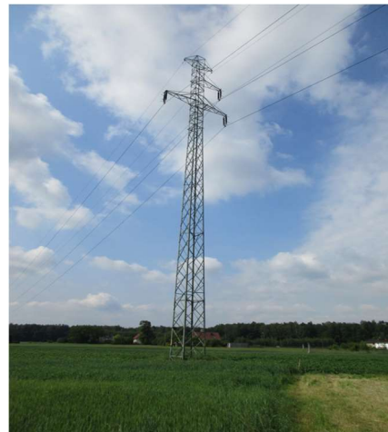
Figure 33 -Damages due to floodplains and subsidence - deviation from verticality (GIG's archives)
