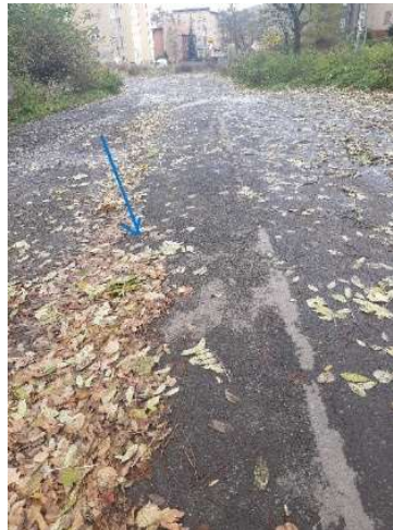
Figure 23 - The example of continuous surface deformation (M.Wysocka)
